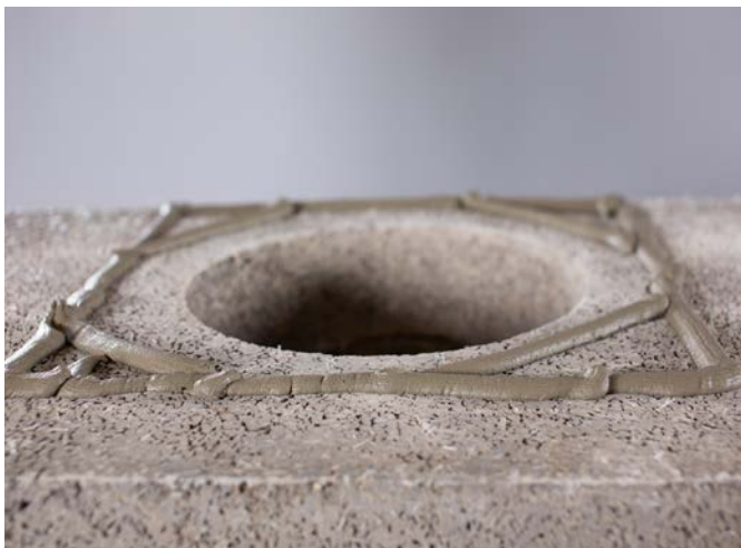
Spread lip glue adhesive in the shape of the chimney block.
