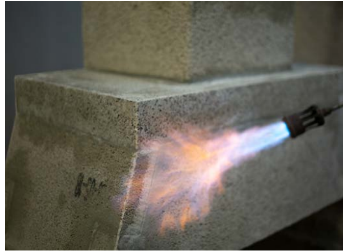
Burn off the fibres on the external surface before rendering.
