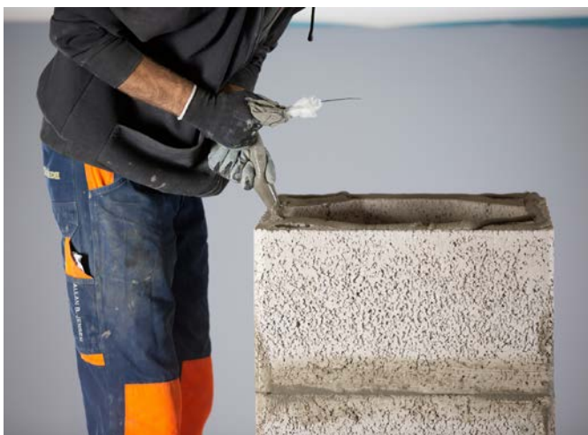
Glue on the next two chimney blocks.
