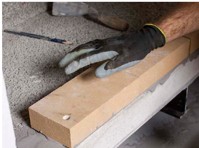
Bed the firebricks on to a 3mm layer of firebrick mortar. Use the tables on the previous page as a guide.
