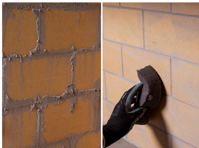
Use the mortar mix to point up the joints between the firebricks once they are all in position. Clean off excess mortar.
